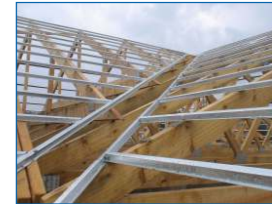
25mm Top-Hat profiles used as tile battens on timber roof trusses.
